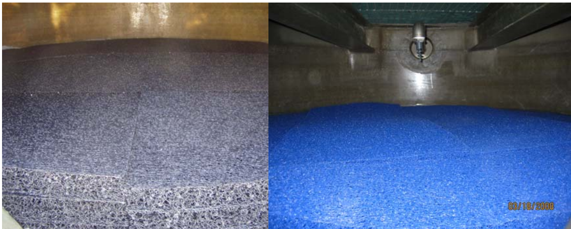
Figure 2. Upper and Lower Media Inside the Vessel
